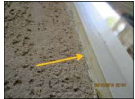
Good sealants around all window perimeters...good.
